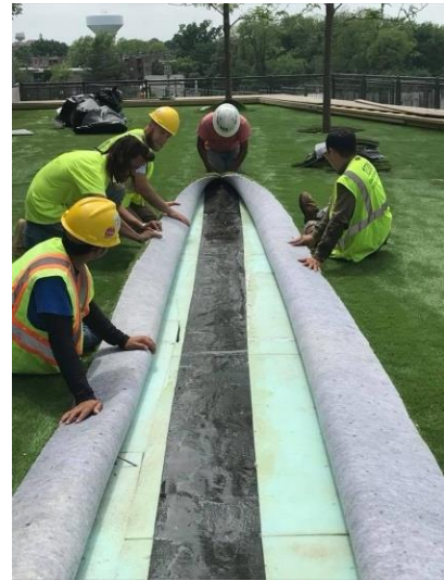
2.0 inch with Turf Installed
