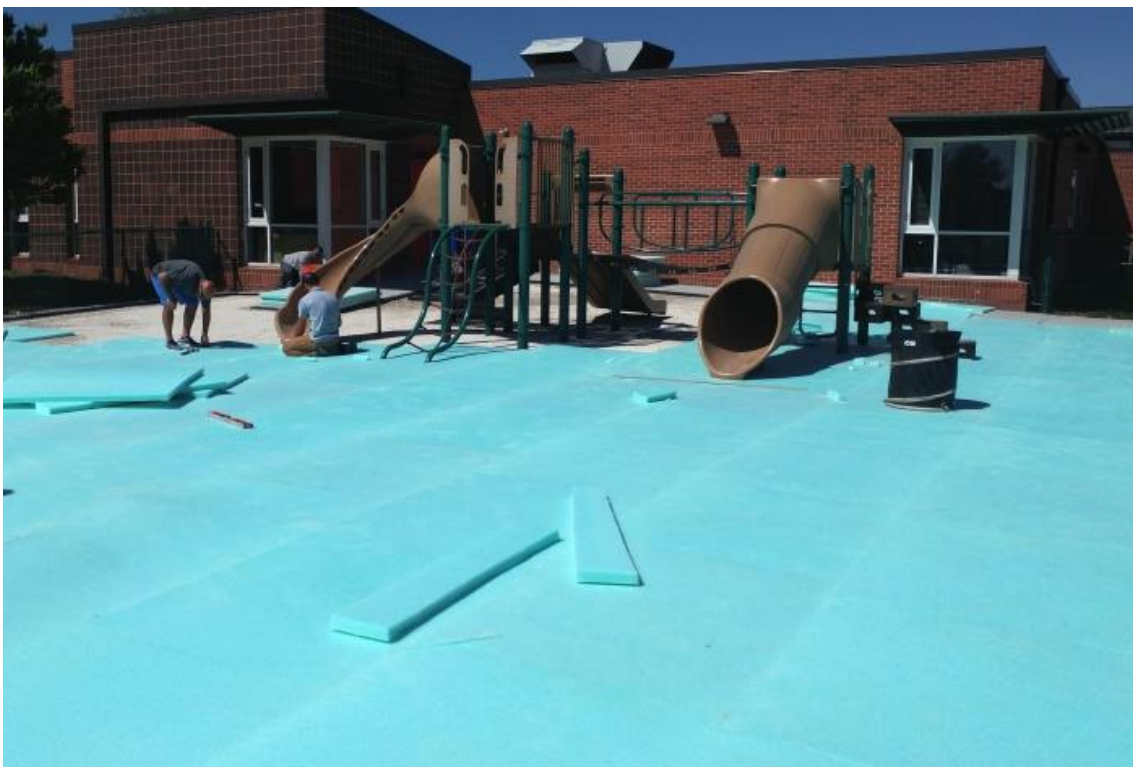
TurfCushion® 2.0 inch installed in Brick Type pattern.
