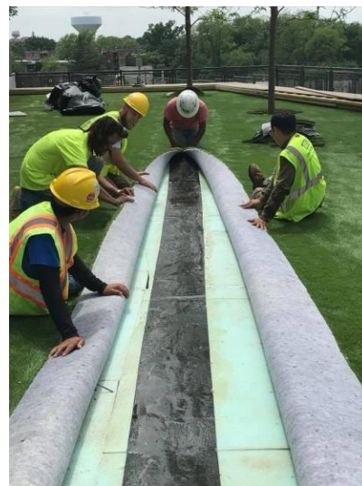
2.0 inch with Turf Installed
